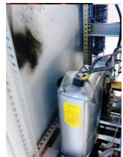
Capacitor damage
