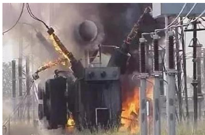
Overheat of Neutral Wire And transformer broken
